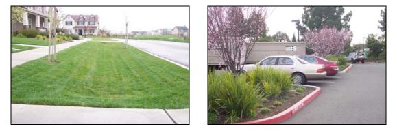
Stormwater management in South Livermore and Palo Alto, California: bioswale for residential neighborhood (left) and pervious surface in parking lot (right).
